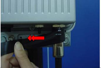
4. Please lengthen the tape before wrapping it around the joint between antenna and N-type connector.
